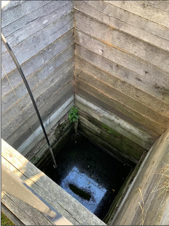
PHOTO: View into the restored cribbed well at Fairbank Oil.
