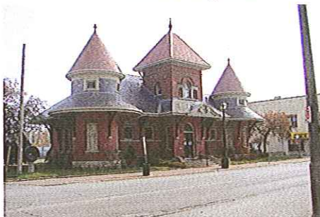
GTR Railway Station, 1903
