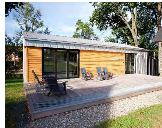
US Green Building Council, Green Education Centre, Baltimore MD
